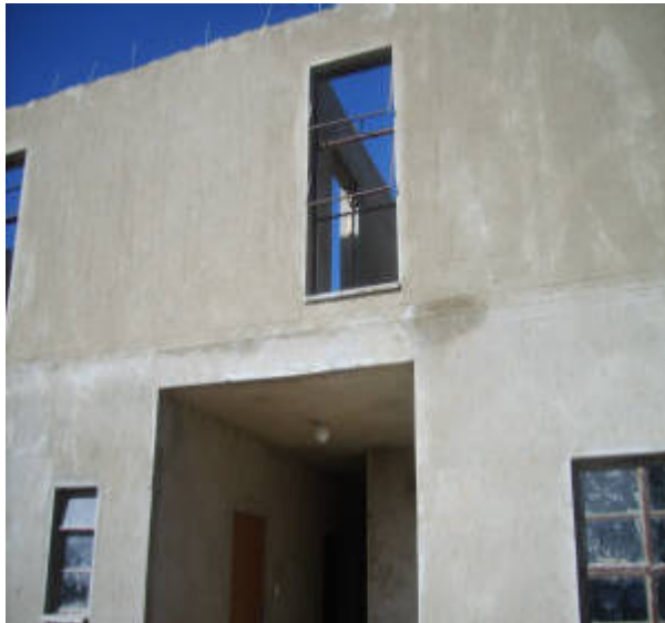
The building grows...
